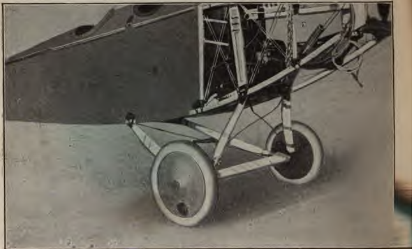
Fig. 100. Landing Gear Installed on Fuselage of Training Biplane.
